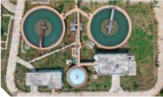
Mega Integrated Rural Piped Water Supply Scheme to 200 MINING-AFFECTED VILLAGES of Hatadihi Block, Keonjhar District, Odisha
