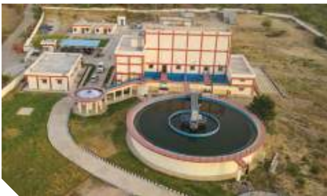
Gulara, Bachouli, and Tilaetha Group of Villages WATER SUPPLY SCHEME IN JHANSI UNDER THE JAL JEEVAN MISSION
